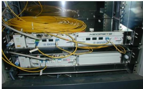
The figure shows the hybrid Raman and Erbium-doped-fibre optical amplifier. Both allow amplifying the optical signal in the fibre without the need for electrical amplification of the signal.
